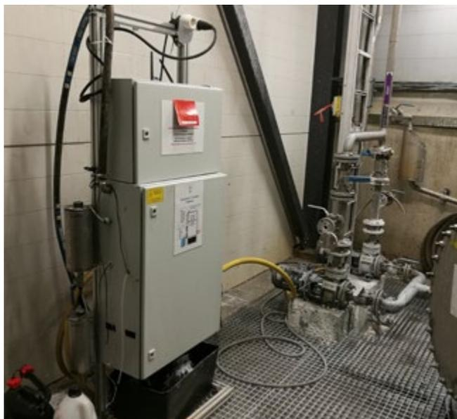
Figure 4.2. Industrial trials of a real-time NIR measuring device developed as part of the BIOMIT project.
